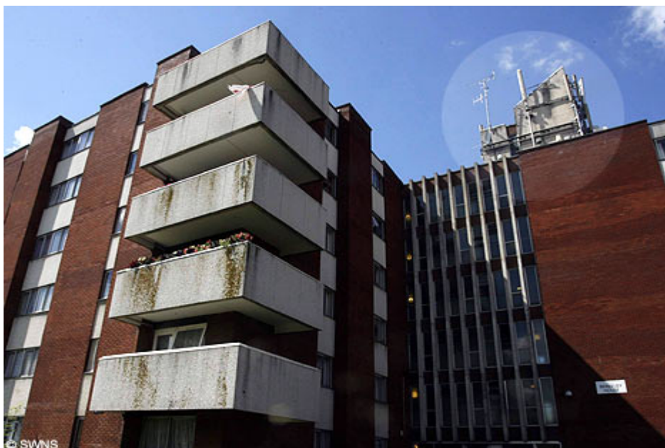
Anger: The mast (circled) on the block known to locals as the Tower of Doom
